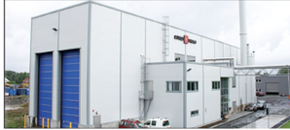
View of Weiss A/S boiler working on solid domestic waste
